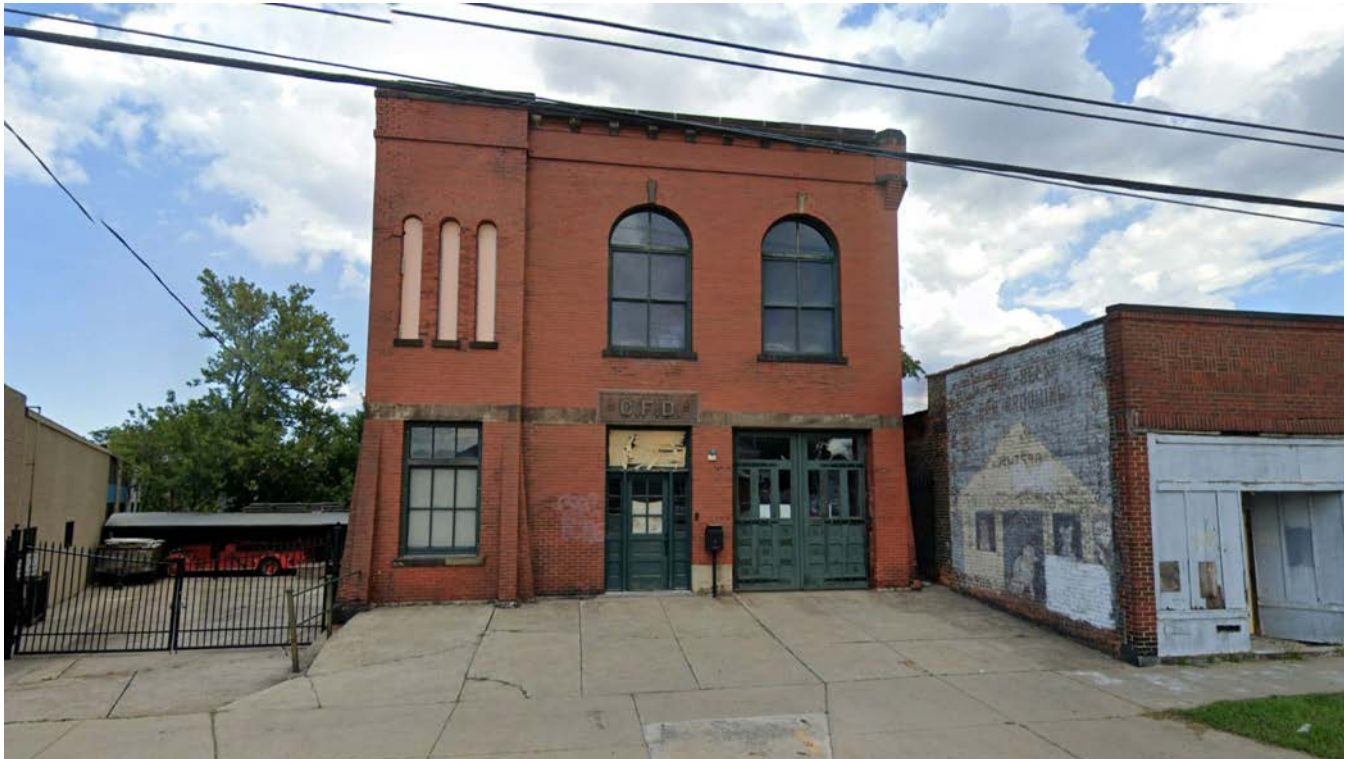
1 Proposed re-use of former fire station as community kitchen
