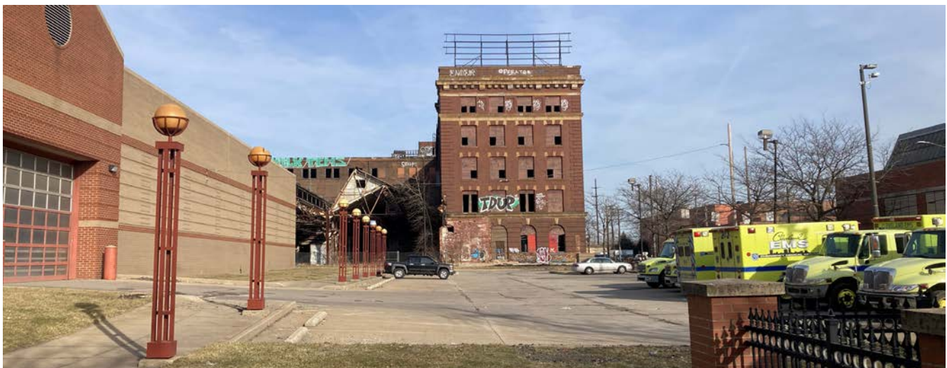
Warner and Swasey Building, Carnegie Avenue, Cleveland
