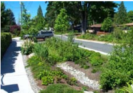
FIG 16 Swale for surface water conveyance. Seattle Public Utilities drainage system project
