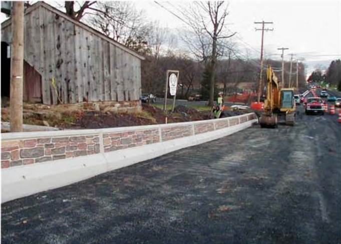
Stone-faced concrete barriers
