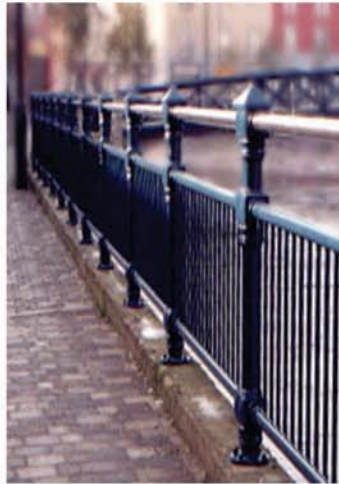
Decorative iron rails
