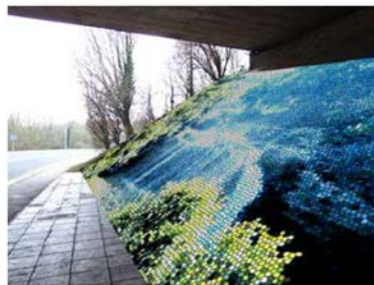
Public art, lighting, and paving would improve the pedestrian connection under the bridge
