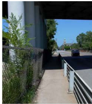
Current conditions under the freeway bridge
