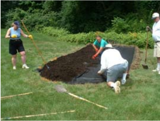
Volunteers working on the construction of a rain garden
